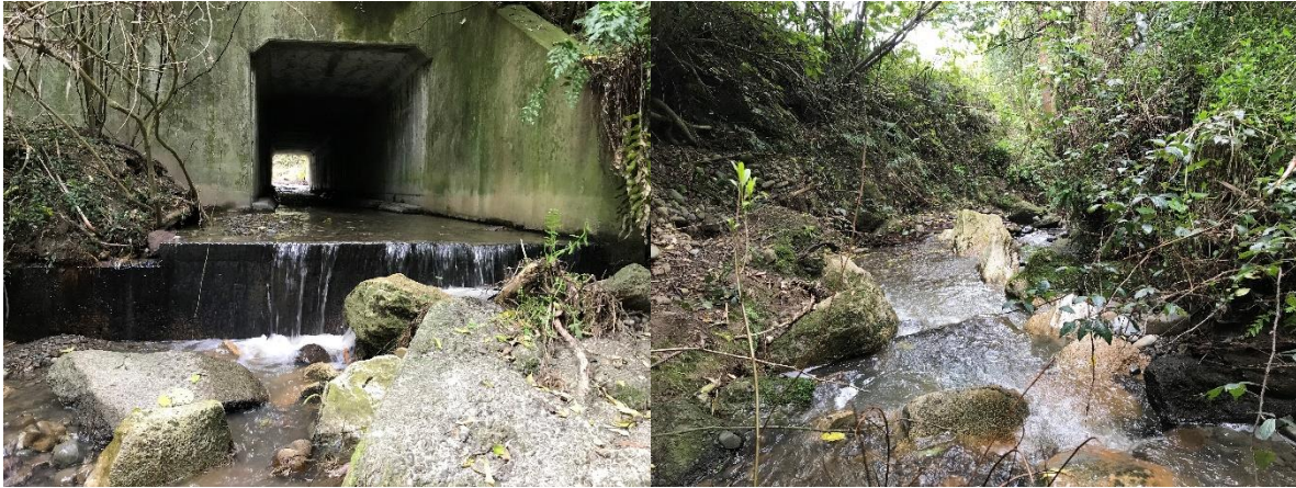
Figure 1: Culvert that runs under the Kiwirail rail line were catchment seven enters the Manawatū River. Photo on the left shows the raised culvert outlet creating a barrier to fish passage for the majority of native fish, Photo on the right is downstream of the culvert looking towards the Manawatū River.
